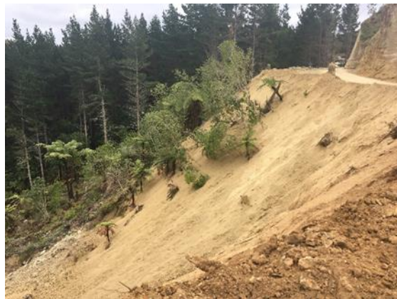
Figure 9 – Side casting of material
