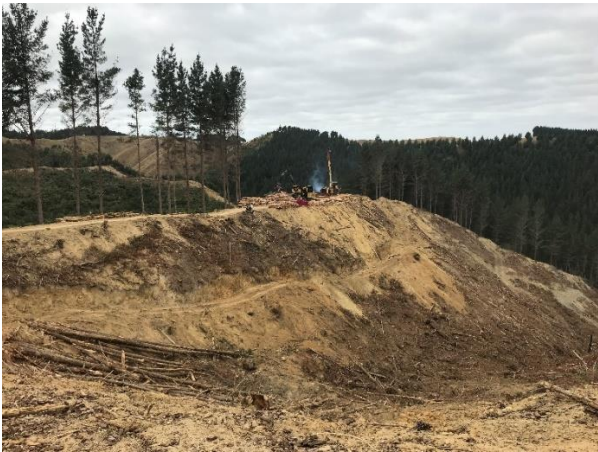
Figure 5 – Poor erosion and sediment controls
